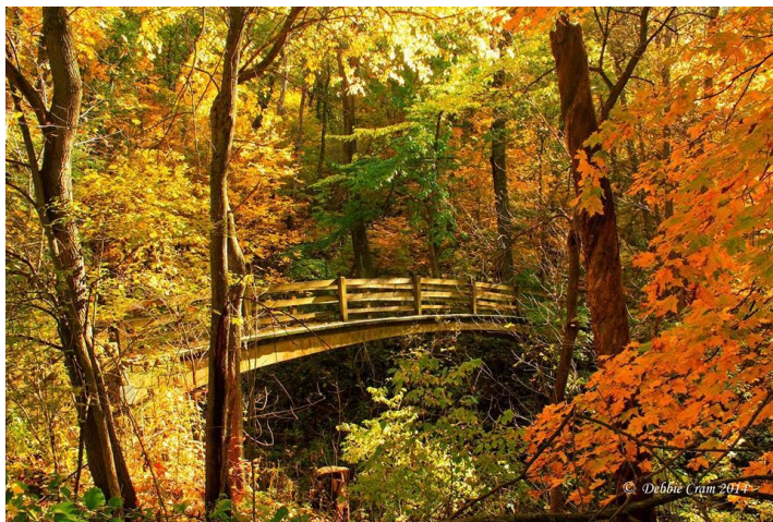
Bridge at Palisades State Park by Debbie Cram
